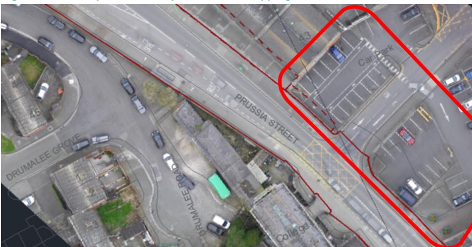
Figure 3.2.86: Existing aerial view at Park Shopping Centre, Prussia Street (Image Source: Google)
