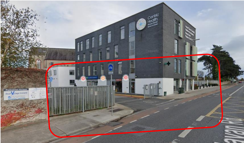
Figure 3.2.78: Existing Street View at Aras Slainte, Navan Road (Image Source: Google)
