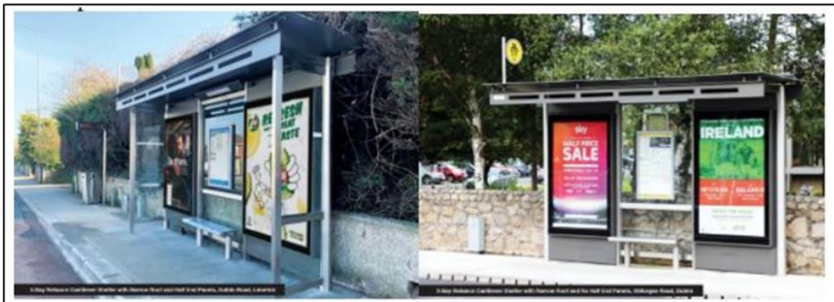
Figure 2.9.7: Example of a 3-Bay Reliance Cantilever shelter with a narrow roof configuration with and without half end panels.
