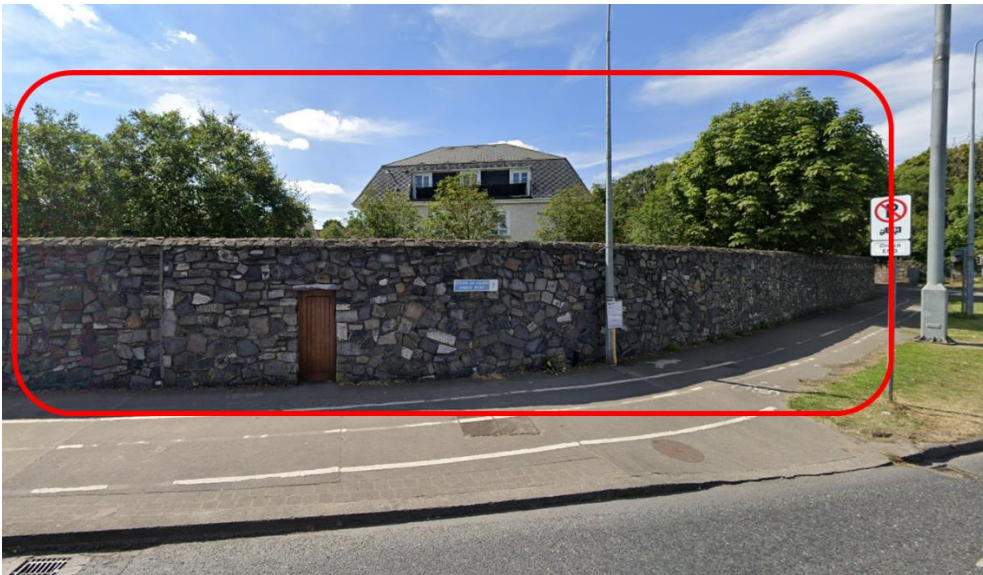
Figure 3.2.44: Existing Street View at Belleville (Image Source: Google)
