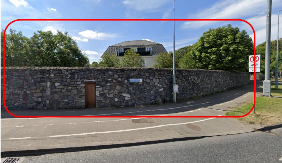
Figure 3.2.35: Existing Street View at Belleville (Image Source: Google)
