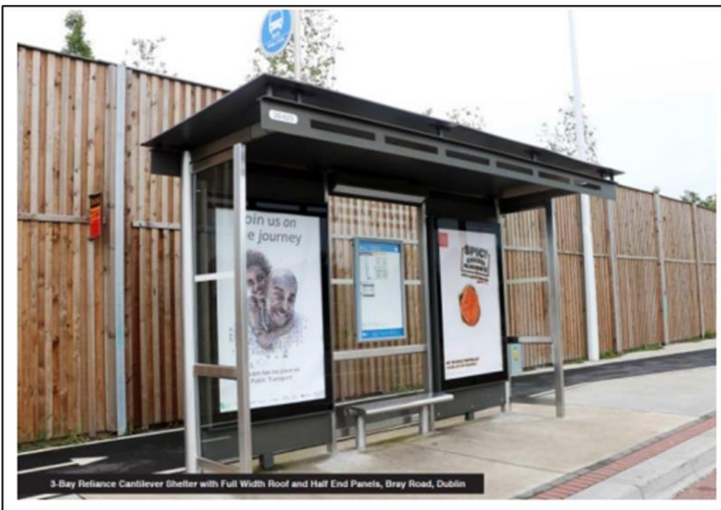
Figure 2.9.6: Example of a 3-Bay Reliance Cantilever Shelter with full width roof and half end panels (source: JC Decaux)
