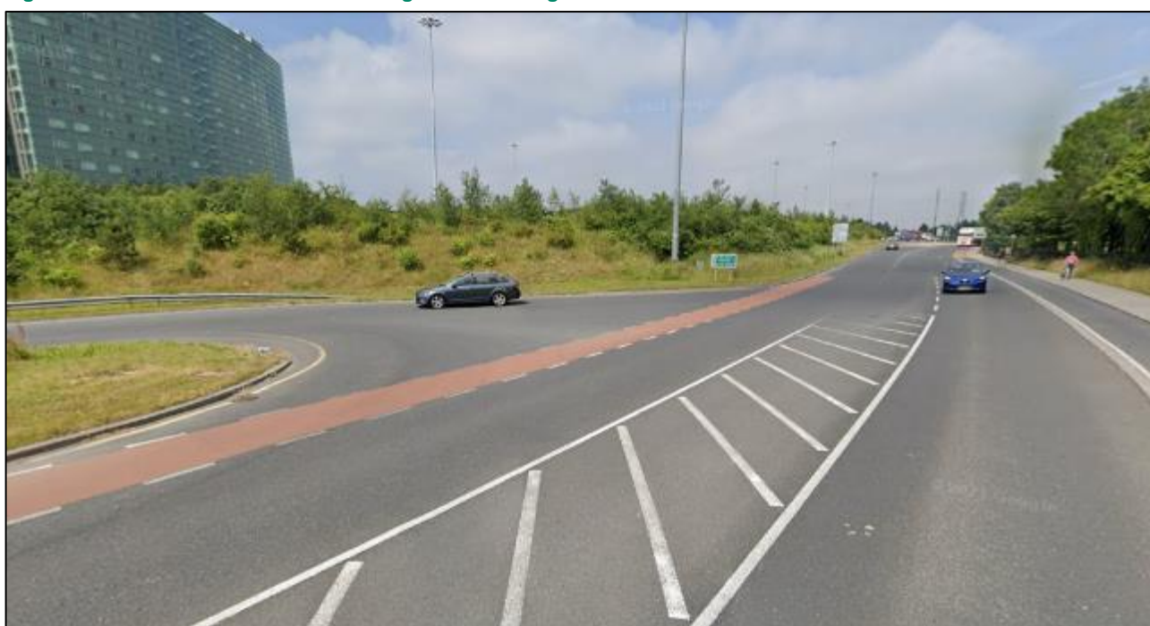
Figure 2.9.44: Streetview image of existing layout at N3 on-slip junction (@2022 google)
